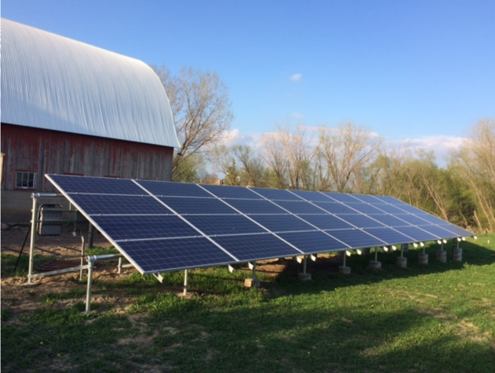
Member's 10.2 kW Solar Installation Stewartville, MN
