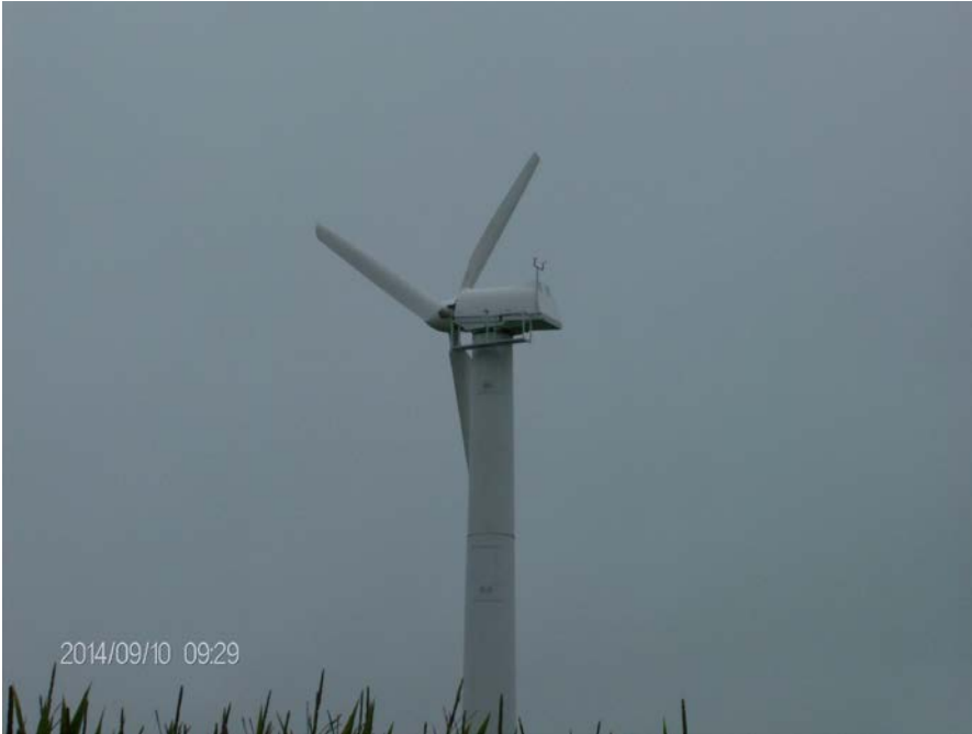
Member 39.9 kW Wind Turbine Elgin Township, MN
